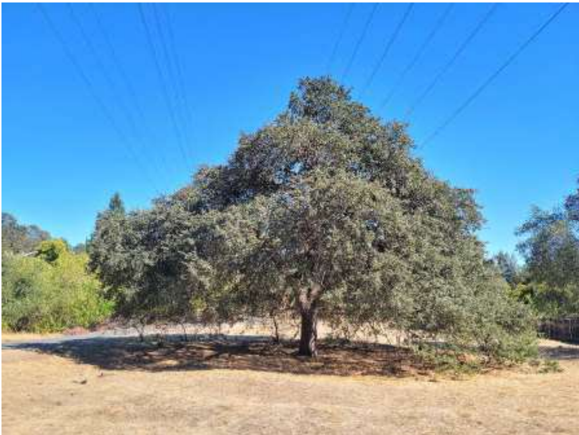
An example of one of the more significant oak trees within the OPTC and the challenges with overhead utility lines.
